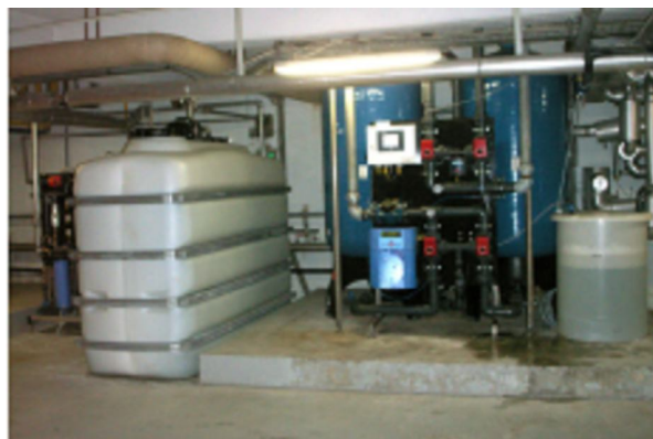
A view of the water treatment plant in the basement below Nordjyllands Regionsvaskeri in Aalborg. To the right is the new HVD softening plant and to the left the RO plant and reservoir tank.
